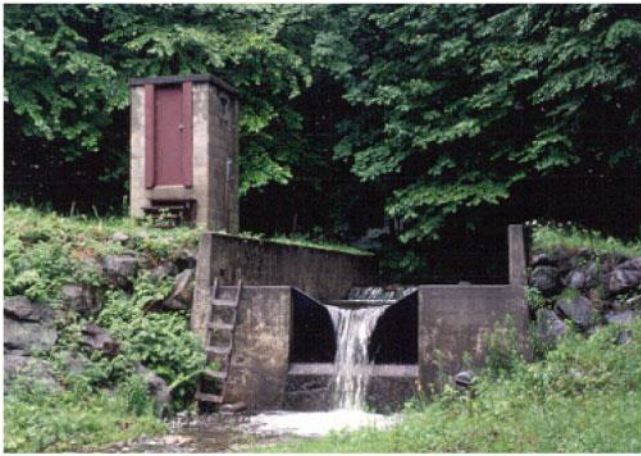
(a) Concrete dam and weir
